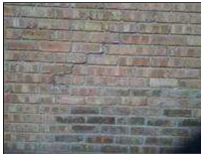
2.1 Picture 1 Masonry Repairs
