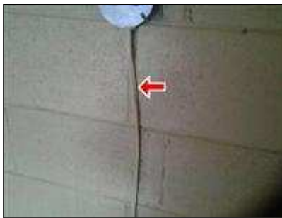
5.2 Picture 2 Romex Wiring to Light
