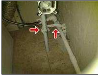
5.3 Picture 1 Ground Bonding Strap and Clamp
