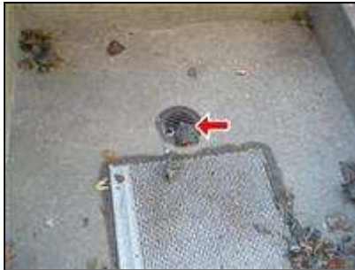
2.5 Picture 3 Areaway Drain
